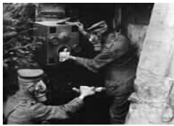
Placing pigeon in cage at trench entrance
